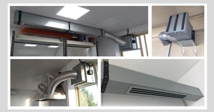
Auxiliary air supply units are intended for use when it is not feasible to introduce the required makeup air through the room ventilation systems.
